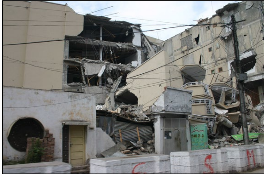
Buildings collapse: scale 10
